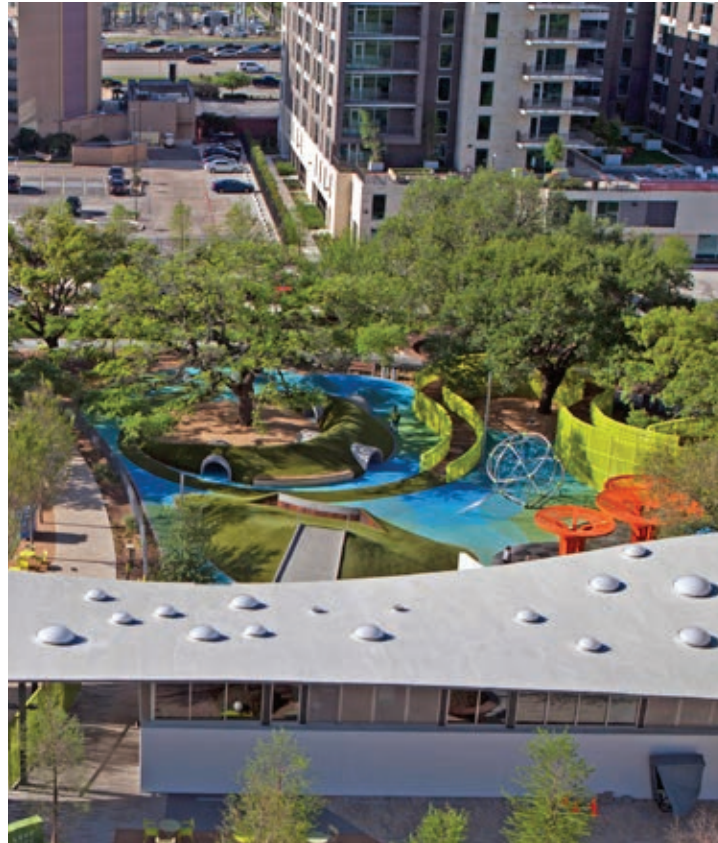
Circular Units, Levy Park Canopy, Houston, TX
