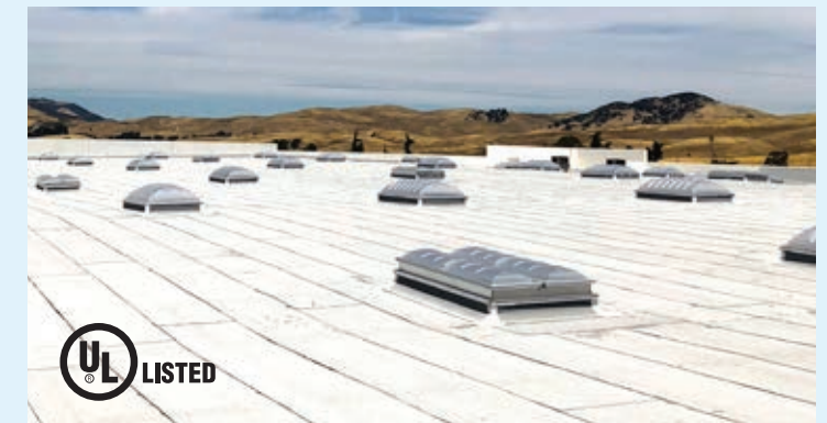
Warehouse, Livermore, CA
