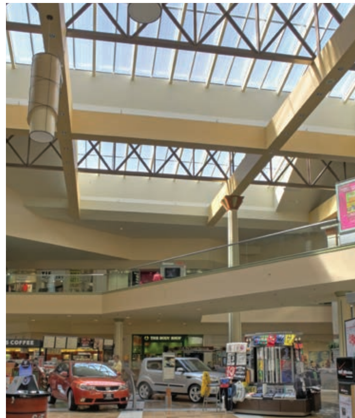
Single Pitch, Rockaway Town Center, Rockaway, NJ
